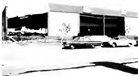
Photo 18. One of three structures in the Bradley light industrial tract that had one or more sections of its walls fail.
